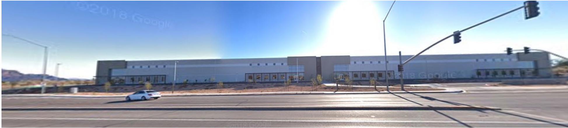
Looking east from Higley Road
